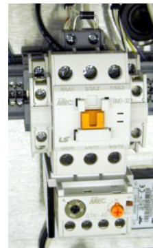
Figure 12. Motor Contactor
